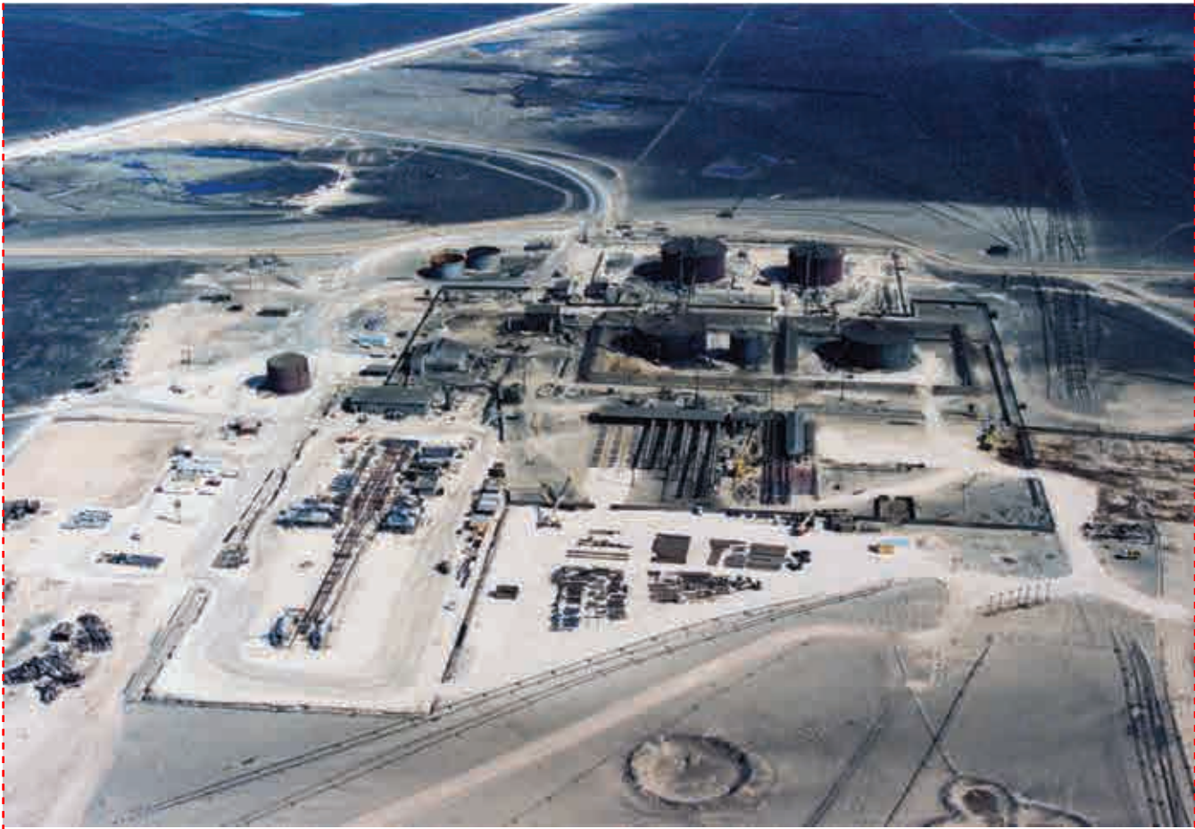
Figure 1.5 Damage to the infrastructure at the Burgan oil fields after extinguishing the oil fires in November 1991
