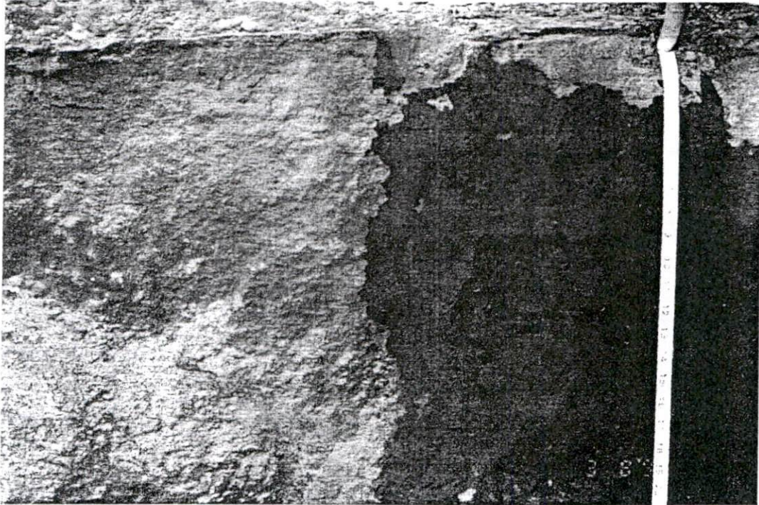
Figure 5a Surface tarimat and slightly oil contaminated subsoil.
