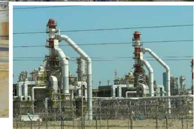
Figure 7. KNPC Shuaiba developed refinery facility (2021)
