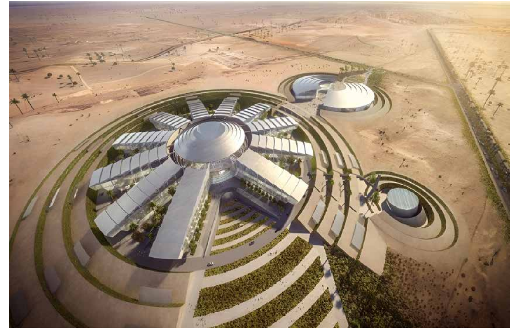
Figure 12. Kuwait International Petroleum Research Center.
