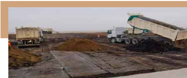
Figure 16. Filling oil sludge after lining SK.
