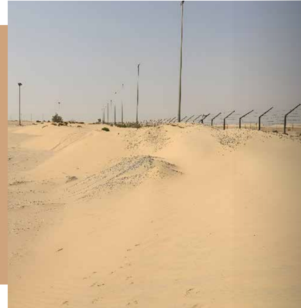
Figure 8. Mobile sand accumulation on depressions, fences, and roads (S)
