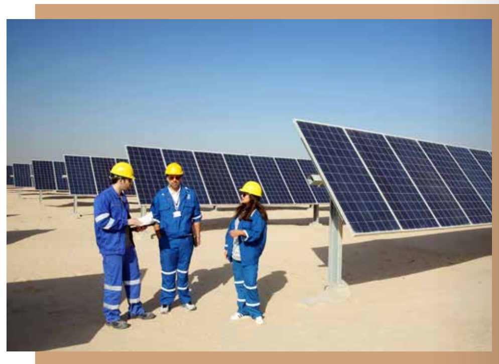
Figure 12. KOC team visiting the solar park in Kuwait.
