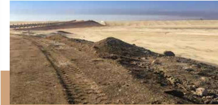
Figure 14. Early stages of landfill construction and filling in the North area of Kuwait (S)
