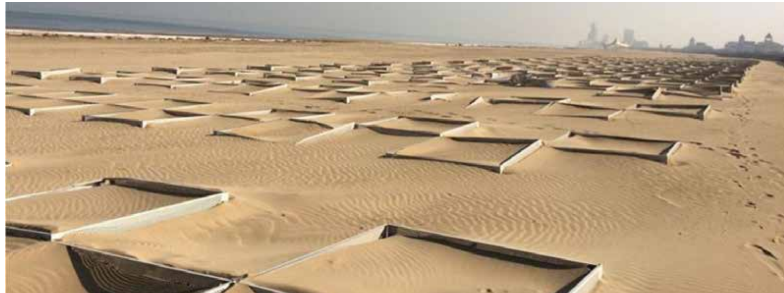
Figure 6. Measures to Control Moving Sand
