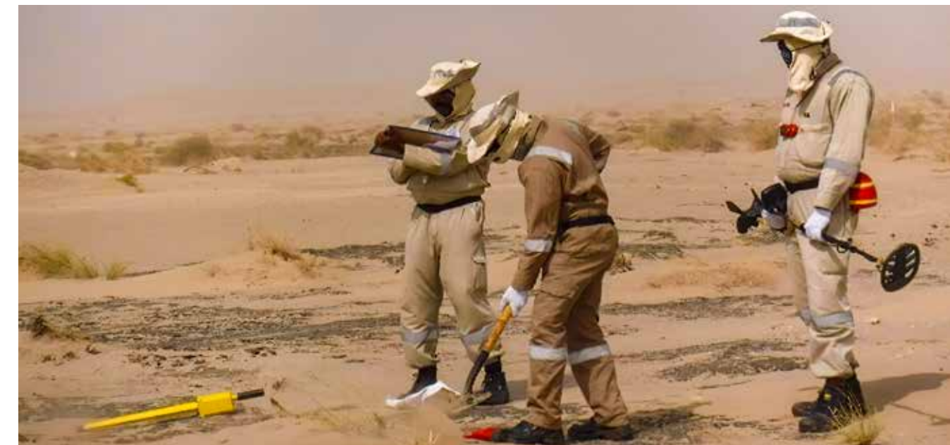
Figure 12. Detection and clearance of UXO in oil contaminated areas prior to soil remediation operations at KOC premises.
