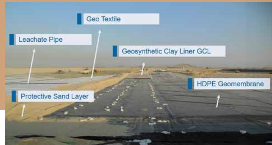
Figure 13. Lining base of Land Fill in the SK Oil production areas.
