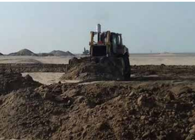
Figure 30. Coastal oil deposit before treatment.
