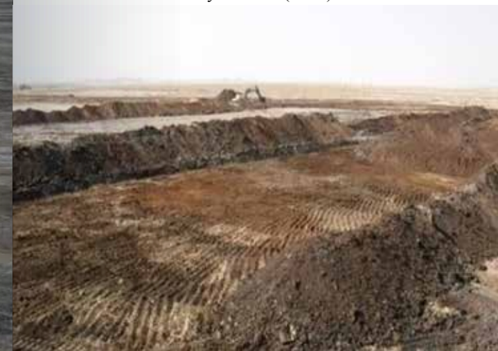
Figure 26. Dry oil lake contaminated area before remediation.
