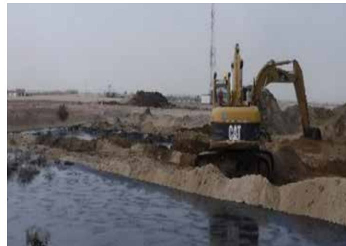
Figure 32. Wellhead pit before remediation
