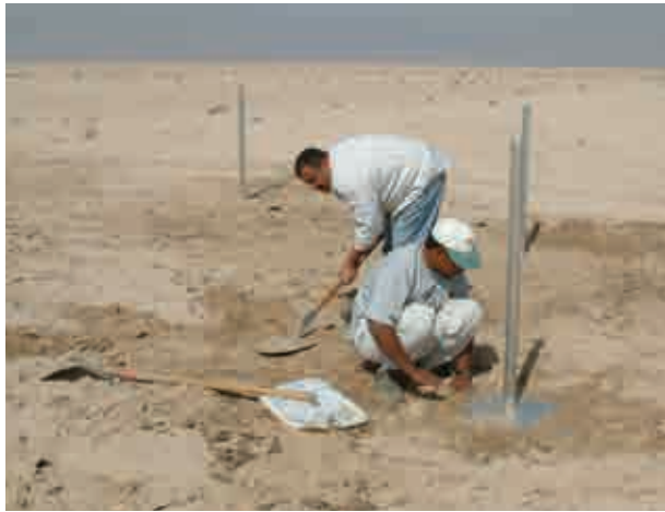
Plate 4. Leveling the ground surrounding the sand traps
