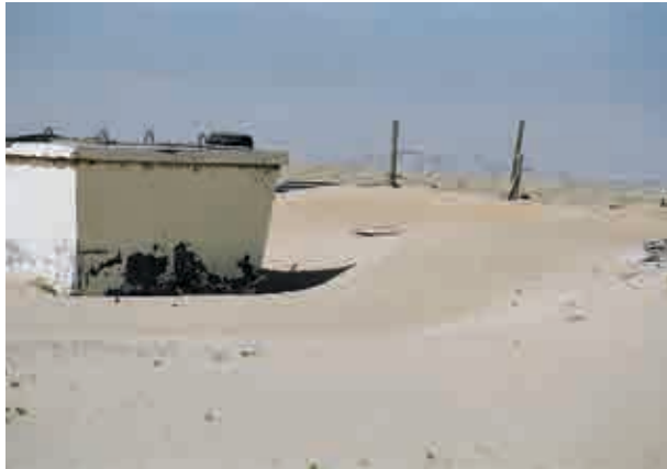
Plate 30. Sand encroachment on ground fortification (June 2003)
