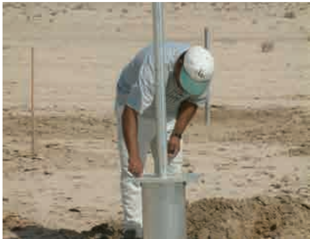
Plate 5. Sand trap installation (station 1)
